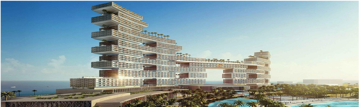
Royal Atlantis Resort and Residence Project
